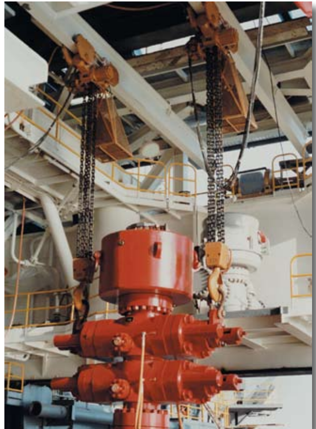
BHS100M (100-ton system) in the process of deploying Blowout Preventer stack
