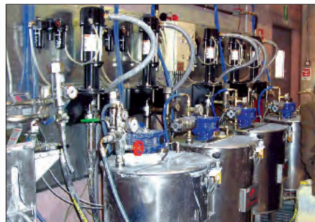
2-ball piston pumps, 11:1 ratio, used in a painting circulating system
